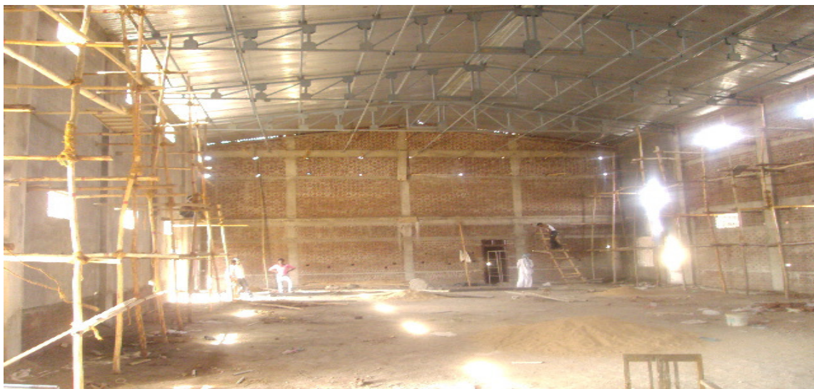
Badminton hall under construction (Interior view)
