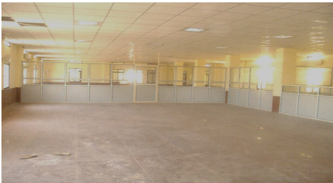
Newly constructed Library building
