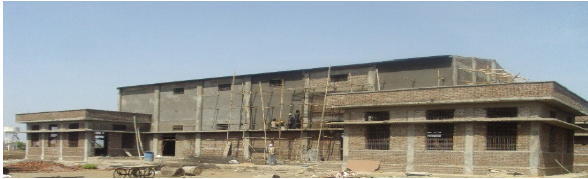
Under construction badminton hall (exterior view)
