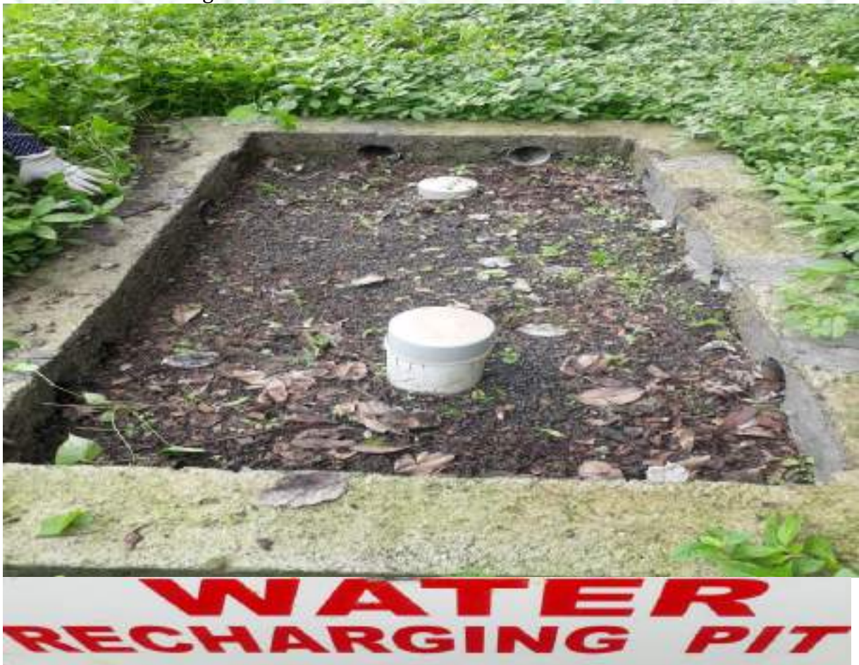
Roof water harvesting has been installed at hostels.
